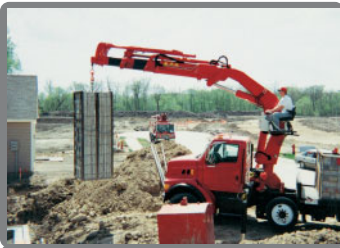
Concrete Wall Construction
